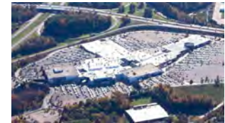
Galleria at Crystal Run Middletown, NY – 1,200,000 sf
